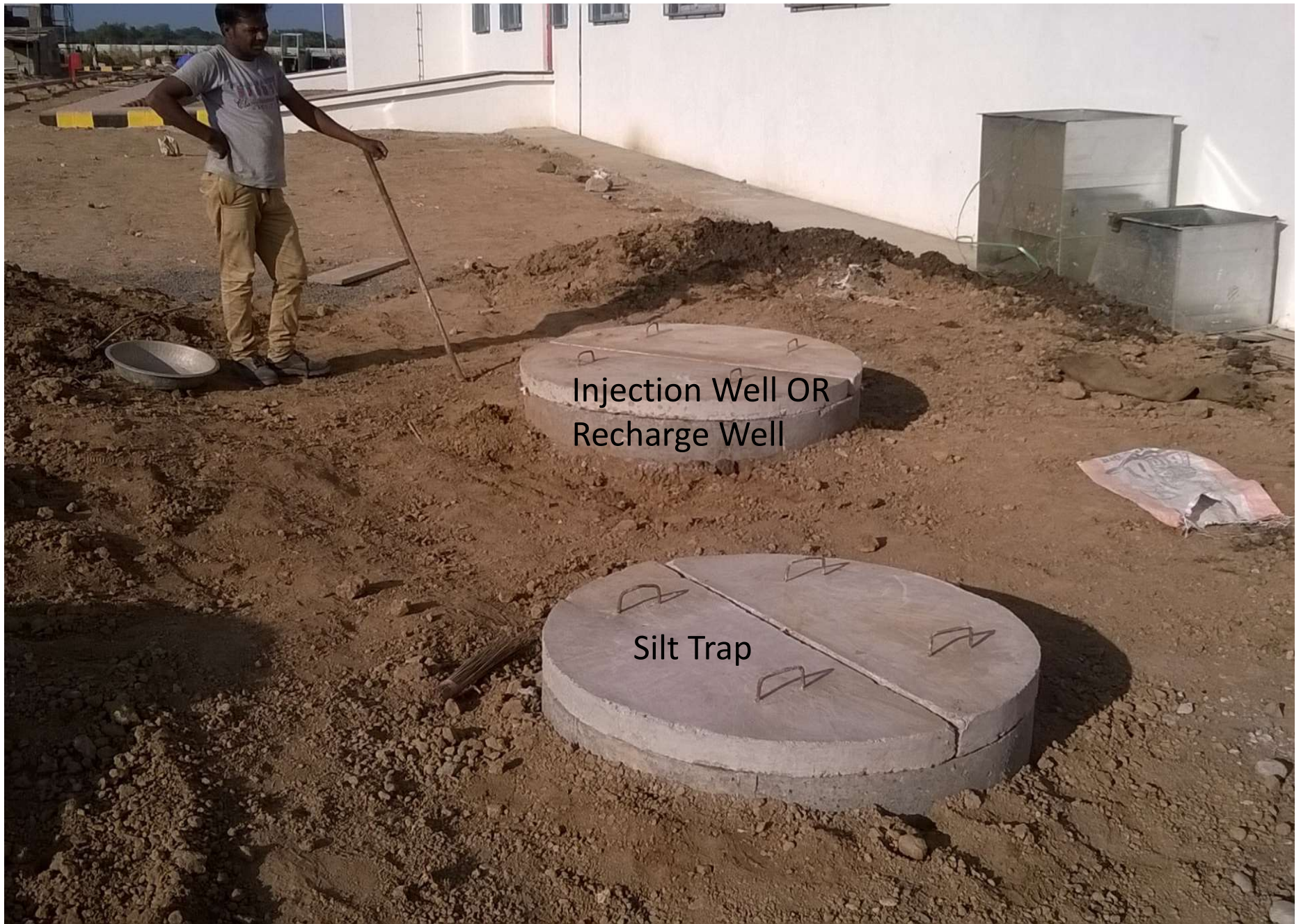
Top View Of Injection Well and Silt Trap
